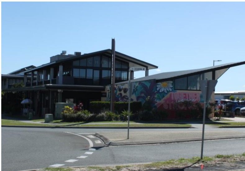
Figure 9: Commercial development to the north-west of the site along Casuarina Way – The Commons
